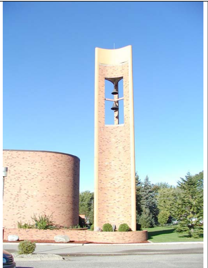
927 E. Old Shakopee Road - Bell tower with hidden T-Mobile antennas, 63 feet tall
