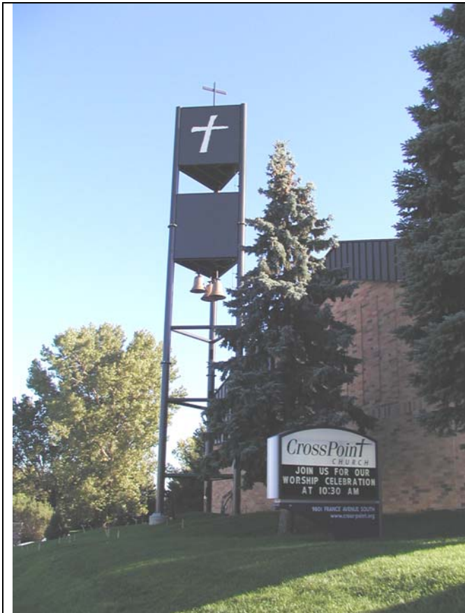
9801 France Ave. S. - Bell tower with hidden T-Mobile antennas, 63 feet tall with cross
