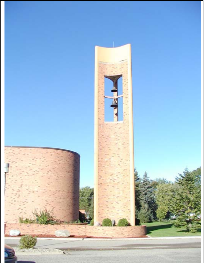
927 E. Old Shakopee Road, Lutheran Church of the Redemption, bell tower with hidden T-Mobile antennas, 63 feet tall
