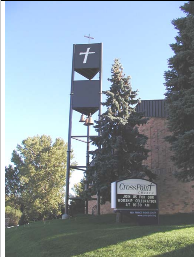
9801 France Ave. S., CrossPoint Church, bell tower with hidden T-Mobile antennas, 63 feet tall with cross
